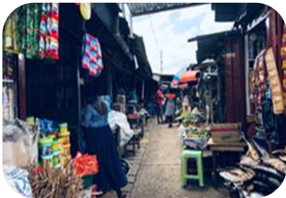
Poor State of Market Structure
