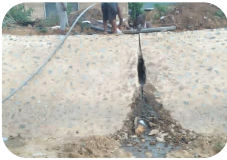
Connection Of Household Sewage Into Drains
